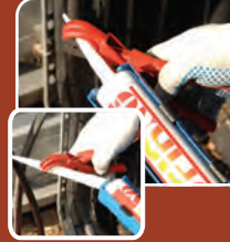
Apply Sufficient Sealant
